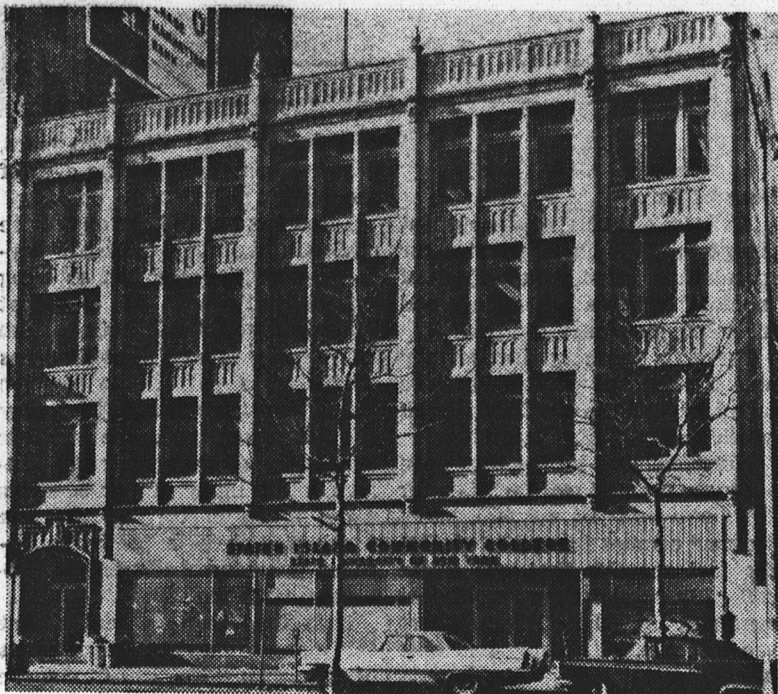
FROM THIS: 50 Bay Street. This unimpressive building has housed SICC for six years. It has been the subject of jokes, curses and exasperation. This "campus" is barely adequate. In approximately two years, its crowded classrooms, crowded hallways, and crowded students will give way . . .
