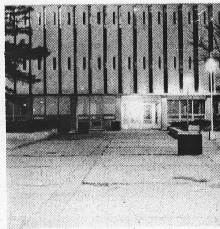
Sunnyside quadrangle is in grave need of renovation.
