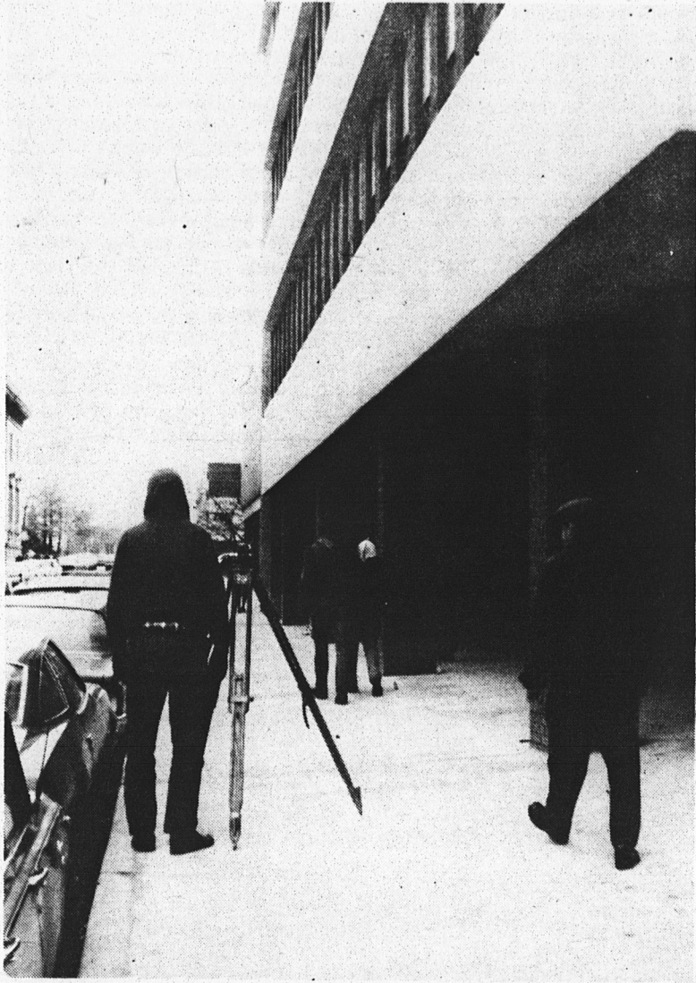
FIRST TWO FLOORS TO BE READY FOR SPRING The 2nd floor will house the Art, Music, and Film Programs, the Guidance and Counselling Masters Program, and the Television Workshop. Two large lecture halls, classrooms, and offices will be located on the 1st floor
