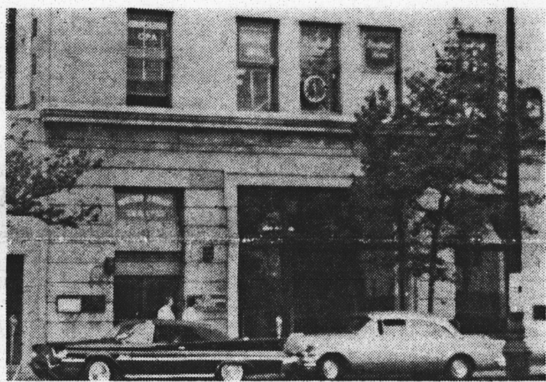
NEW LIBRARY — 28 BAY STREET
