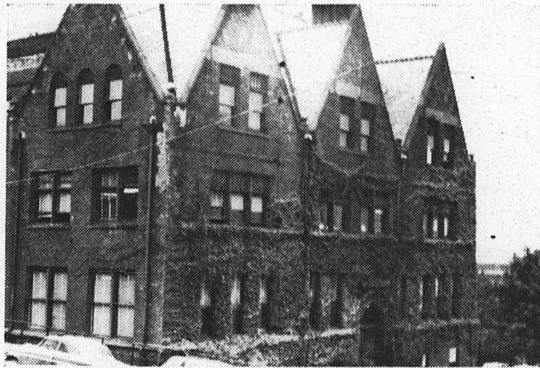
ACADEMY BLDG.: Ivy covered main entrance on 45 Wall Street.
