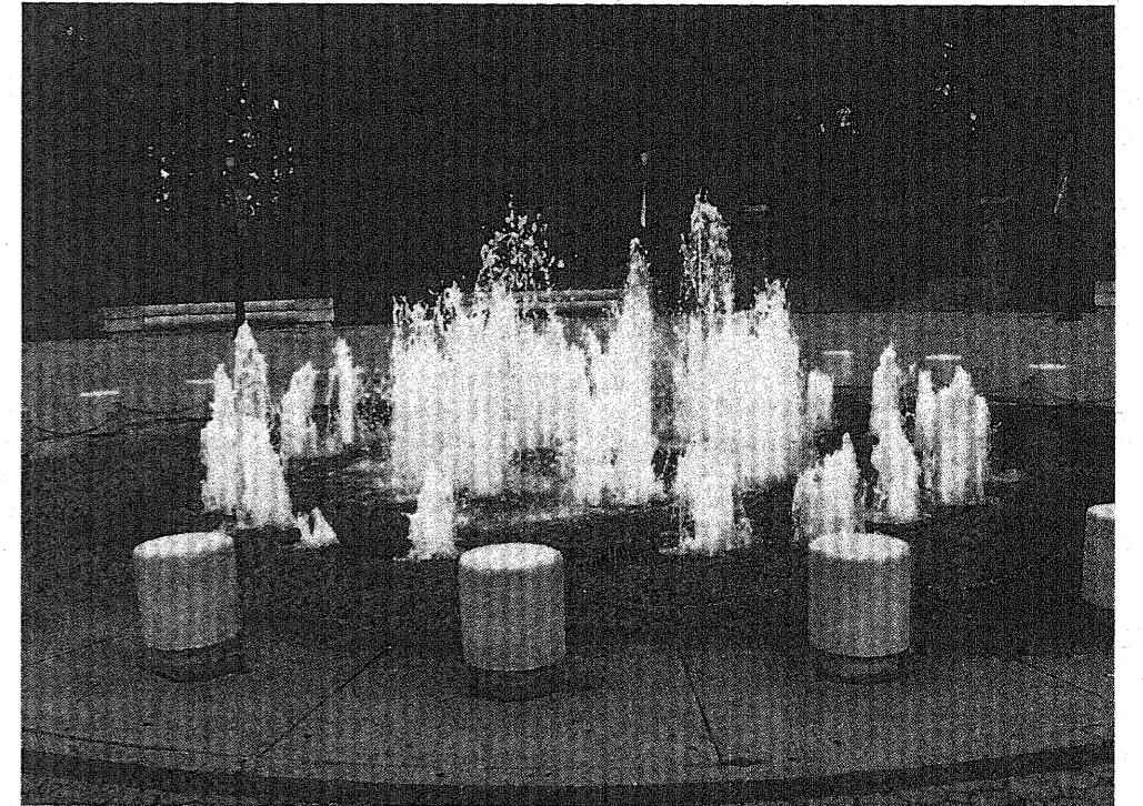
The fountain behind the 1P building is in disarray. The decorative pillars and the water streams are uneven on top of the poor drainage.
