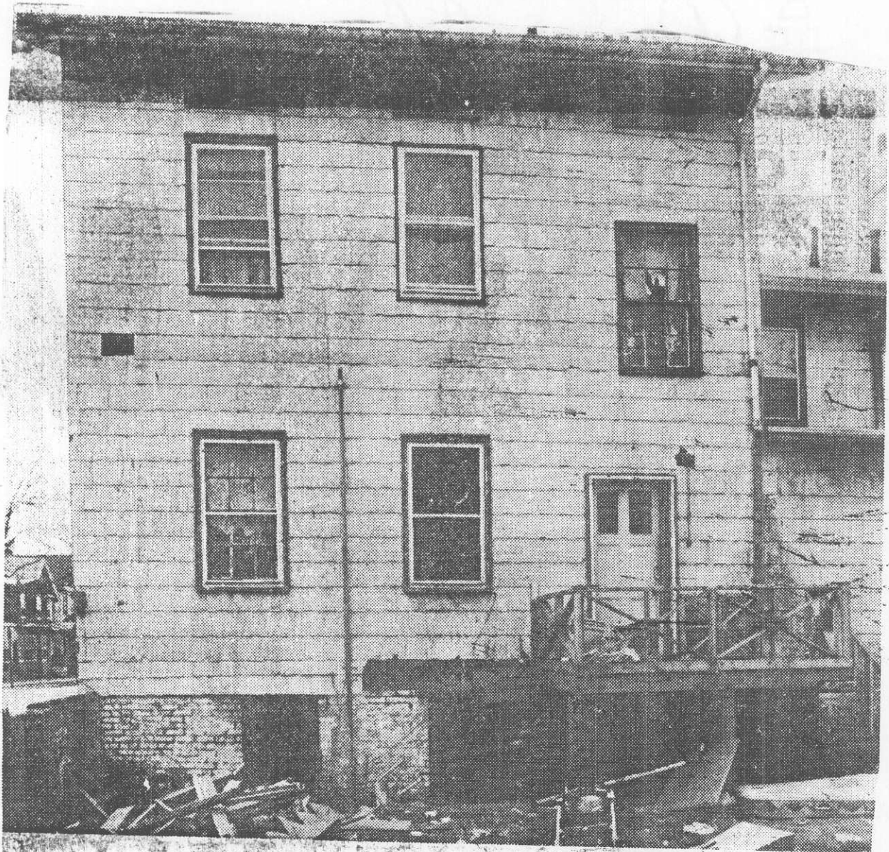
Debris litters the backyard of the dilapidated single-room-occupancy residence.
