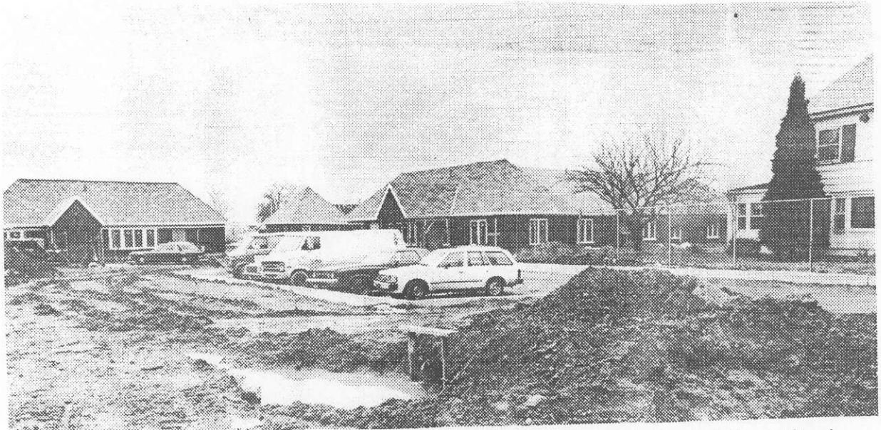
The complex is served by a new roadway and was located to avoid the nearby Corson's Brook Woods area.
