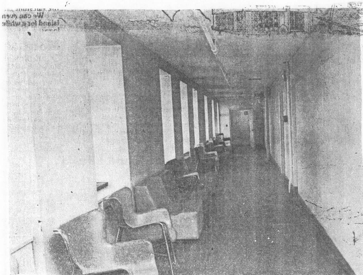
The interior of Building 2 at the SIDC — the center's largest building — shows the need for renovation.
