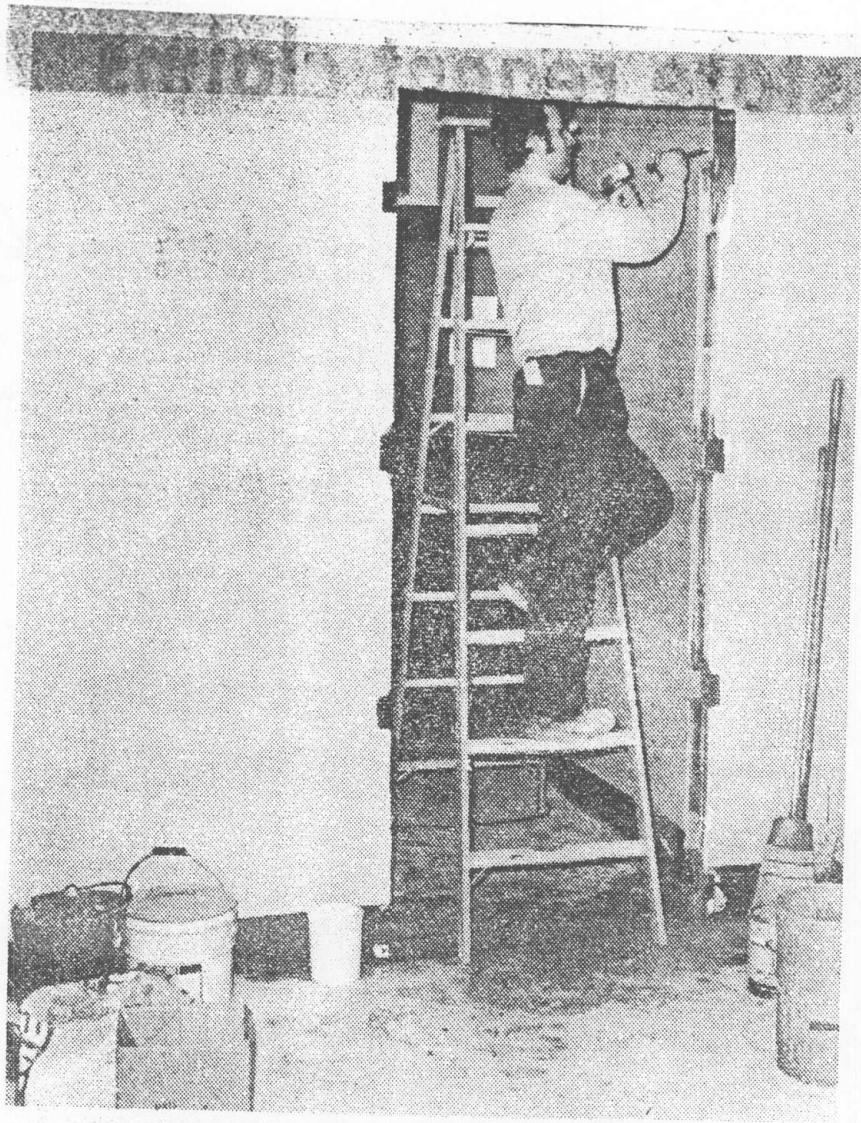
A workman frames out a doorway area in the new office complex of Assemblywoman Elizabeth Connelly at Willowbrook Developmental Center. The Democratic lawmaker is scheduled to move from her West Brighton office next month.
