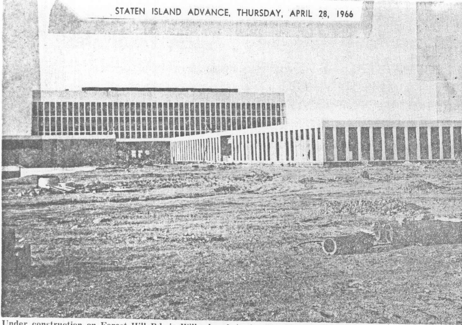
Under construction on Forest Hill Rd. in Willowbrook is the $7-million Institute for Basic Research in Mental Retardation.
