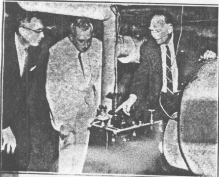
William Musicus (l.), executive director of the New York State Mental Hygiene Facilities Improvement Fund, and Dr. Jack Hammond watch as A. W. Banks (r.), area engineer for the Department of Public Works, explains function of new water valves installed at Willowbrook State School.
