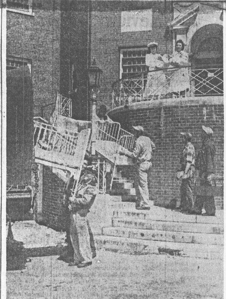
Workmen move cots into the main medical building—formerly the large central building of Halloran VA Hospital—at Willowbrook State School in conjunction with movement of 200 patients into the reactivated wards.
