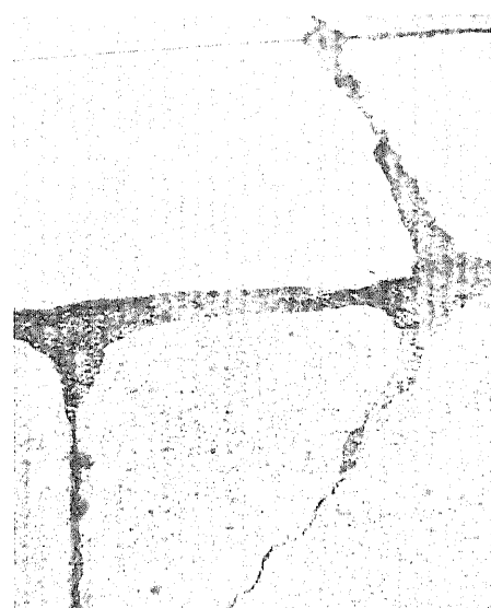
Cracks in the campus walkways are often large enough to get a foot caught which could result in tripping or falling
