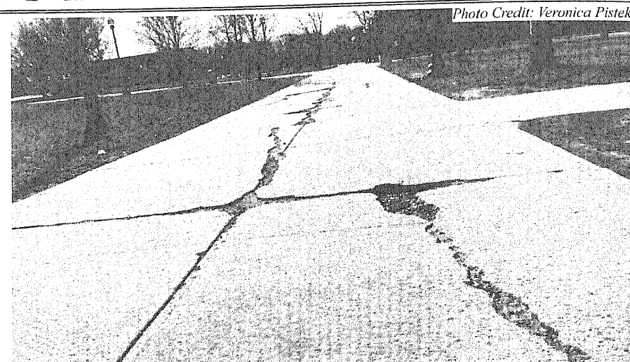
The cracked and rugged sidewalks are not safe for mobility. Handicapped people currently have minor issues.
